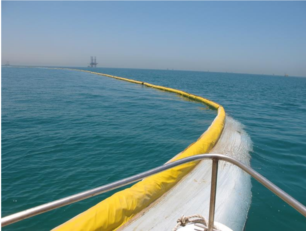
Figure 2. A view of the deployed silt curtain around the trenching site in Safaniyah
