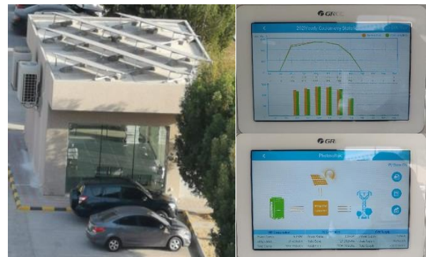
Solar PV roof top air conditioned Bus-Stop in the KFUPM campus (left) aided with smart meter (left)
